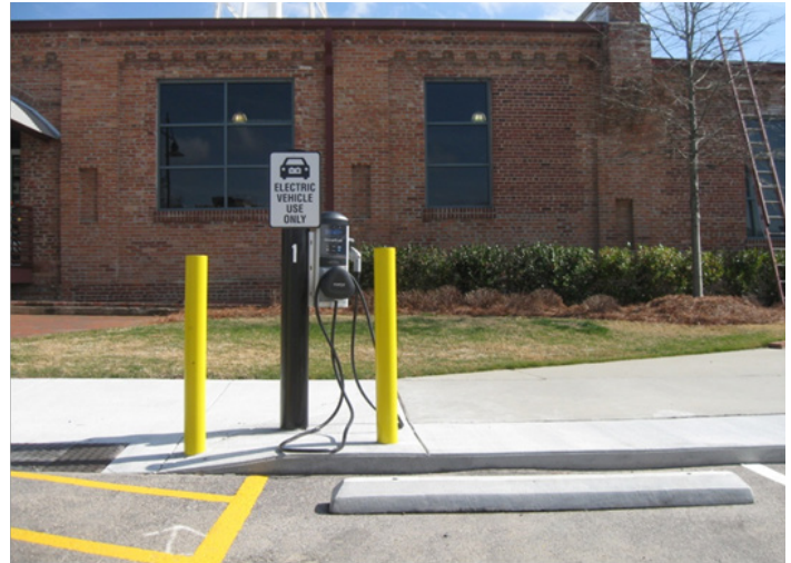
Figure 3. Over-protection can hinder accessibility of charging stations.
